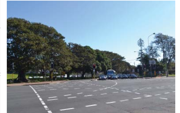
Figure_1.12. Cleveland/South Dowling Street intersection
